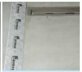
**11** Waterproof all the joints using waterproof tape and waterproof corners then fit the decorative grate, having first inserted the hair trap.
