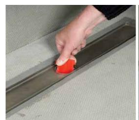
**9** Screw the flange ring through the Showerlay into the drain below. Hand-tighten using the red "key". No sealants should be used.
