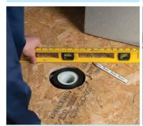
**5** Ensure that the floor is level and clean. Using a cement-based flexible tile adhesive, stick the Showerlay to the floor and position the drain tray into position.
