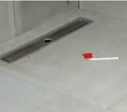
**10** Showerlay-Linear are 40mm thick. The rest of the floor can be raised to this height using Multiboard 40mm.
