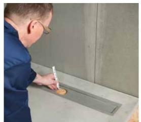
1 Decide where the Showerlay is to go, then mark out the position of the drain hole.
