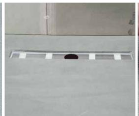
7 Stick the four 4mm self-adhesive pads to the metal base of the Showerlay.
