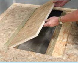
**B** Make support shelves with the cut up flooring and battens fixed to the side of the joists.
