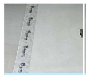
**9** Use Marmox Self-Adhesive Waterproof Tape over all the joints with the surrounding floor and walls. Waterproof corners may also be used.
