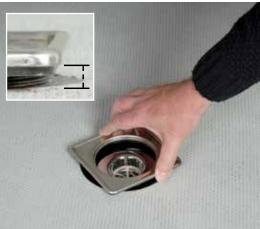
**10** Twist to align the height of the frame with that of the tiling. For thicker tiles, use the clip on extension to the black thread but DO NOT USE on tiles thinner than 10mm.
