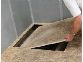
A Decide where the Showerlay is to go, draw around it and cut the floor section out using a jigsaw.
