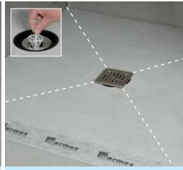
12 There is no need to prime the unit, simply tile with cement-based tile adhesive. If tiles are greater than 10cm, they should be cut along the lines shown.
