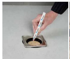
Decide where the Showerlay is to go, then mark out the position of the drain hole.
