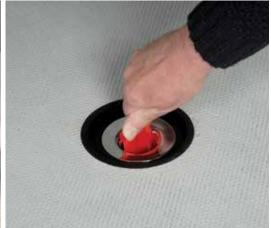
7 Screw the flange ring through the Showerlay into the drain below. Hand-tighten using the red "key". No sealants should be used.
