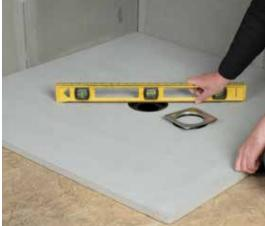
**6** Using a cement-based flexible tile adhesive, stick the Showerlay to the floor, checking again that it is level.
